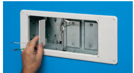
4 Install voltage separator.
