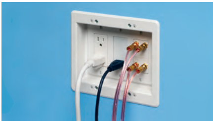
4 Install devices, then the wall plates.
