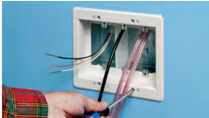
2 Pull cable. Insert box in hole. Tighten mounting wing screws to hold box securely against wall.
