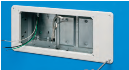
3 After drywall is installed, add trim plate, then install enclosure assembly to the wall with outer screws.
