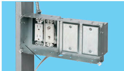
1 Attach box to steel stud using #6 screws. Pull wires.
