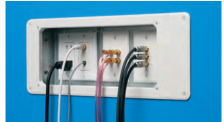
5 Install devices and plates.
