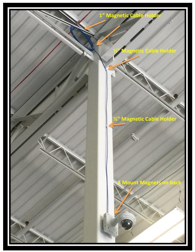
Easiest, Fastest, Install. No Drilling Required. UL Listed and Plenum Rated.
